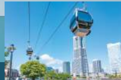
1 YOKOHAMA AIR CABIN (約2,600m)
